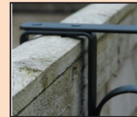
These simple brackets can be also adapted to act as temporary brackets as shown here. This one can hook over fence panels
