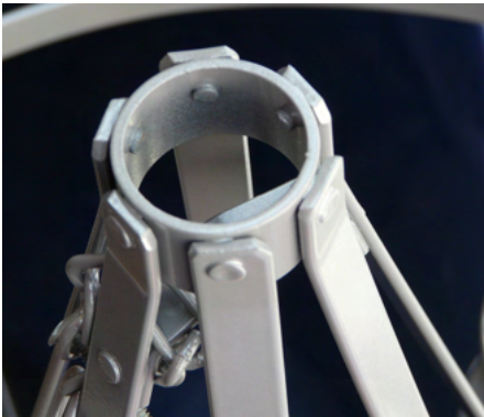
Collar with riveted end fixing.
